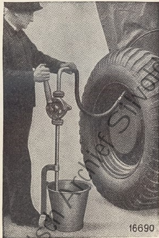
Fig. 91: Water in de band pompen
